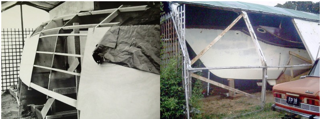
Plywood being applied. Cabin being built.
