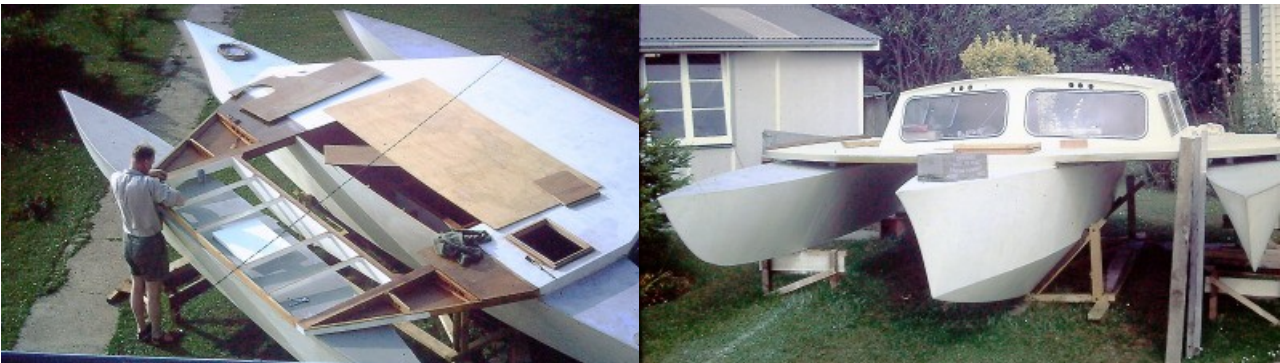
Constructing the deck and the cabin.
