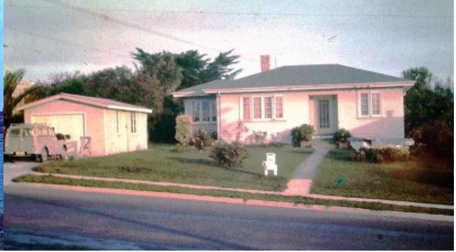
34 Esmonde Rd with the new garage.
