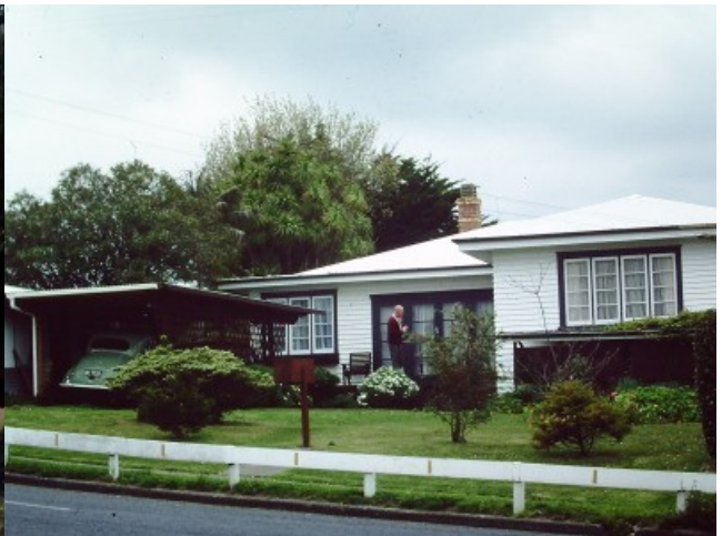
The extensions, car port and boat shed.
