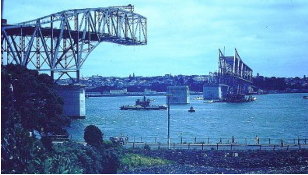
Harbour Bridge with piggyback section.
