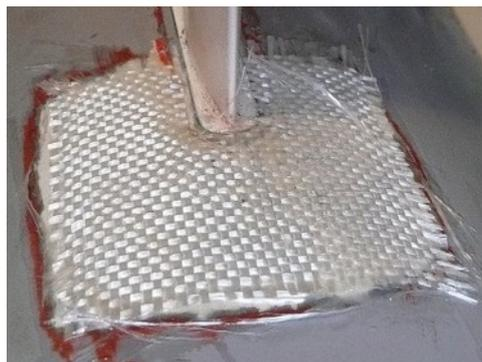
area. A patch of glass fibre was pressed down over this to hold it in position. When dry I added further coats of epoxy.
