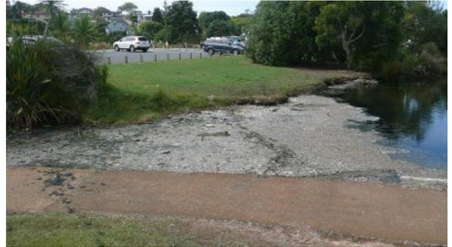
On Wednesday 20<sup>th</sup> I visited the pond and contractors had been working to empty the forebay. Apparently 7 truckloads had been removed at that point. The temporary dam had failed and they were pumping the water out again (photo below) so that they could put a camera through the culvert pipe that runs under the road. The forebay is now about 4 feet deep.
