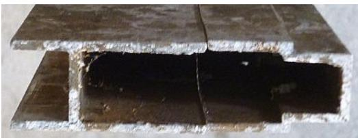
The weir gate boards are aluminium extrusions that clip together. Each board raises the level by 3 inches (75mm).
