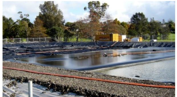
While the dredging was being done the silt bag inflated to the level of the bund rim. It has since subsided as it de-watered.
