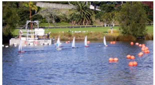
Dredging has started. The raft was moored on the far side with the silt pipe, supported by orange buoys, ran across the pond cutting it into two parts. The white buoys supported the power line but these were well out of the way.
