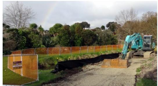
Work continues slowly on the main pond. A digger has been moved to the 'Eastern Stormwater Drain' to clean it out and to construct a forebay which will catch the silt before it gets into the pond. Forebays will also be constructed at the North end of the sailing pond and on the Western Arm.
